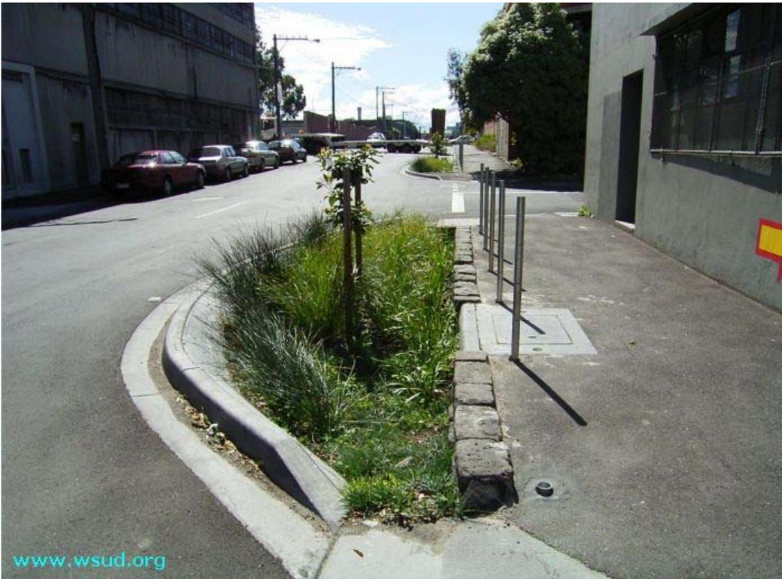
**Plate 1.6 Bioretention pod in road**
