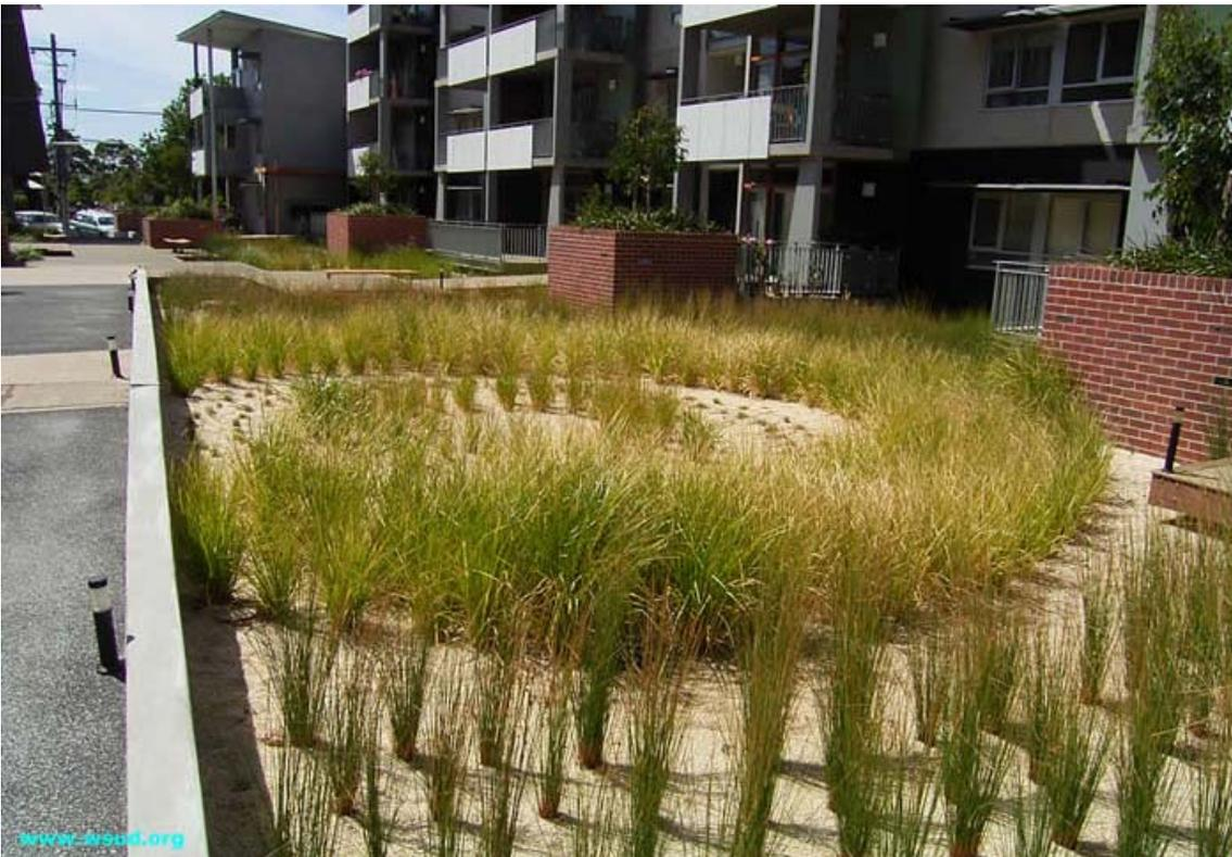
**Plate 1.5 Bioretention basin in medium density development**
