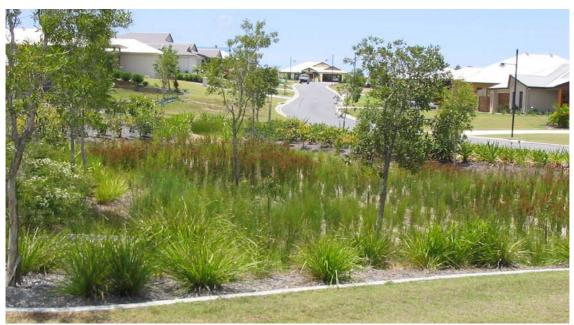
Plate 1.1 Bioretention basin in a streetscape setting
