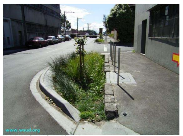
Plate 1.6 Bioretention pod in road
