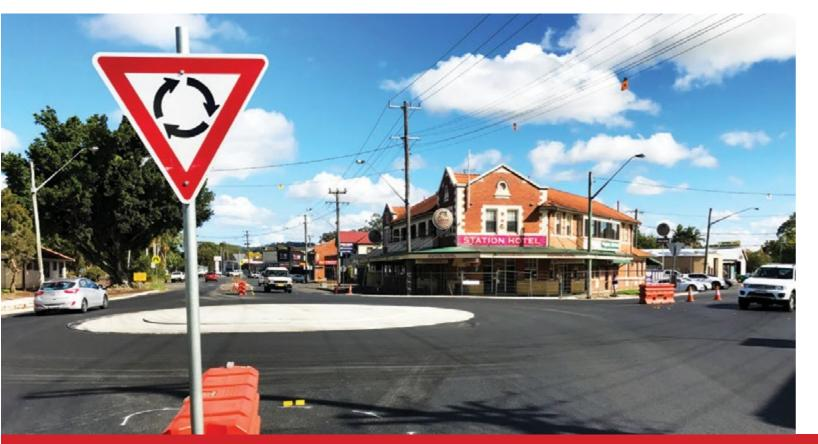
Pedestrian accidents were recorded at this site and the roundabout has been designed to improve pedestrian safety through relocation of pedestrian crossings as well as new median strip fencing outside the Union Street shops to encourage people to use the safer pedestrian refuge points.
