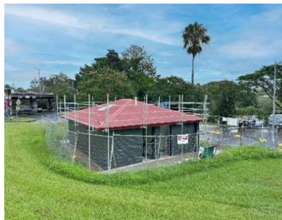
Riverside Park Toilets
