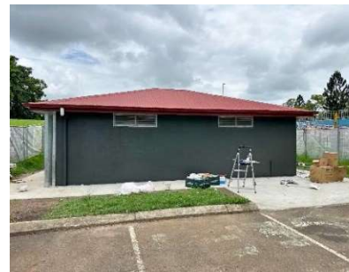
Riverside Park Toilets
