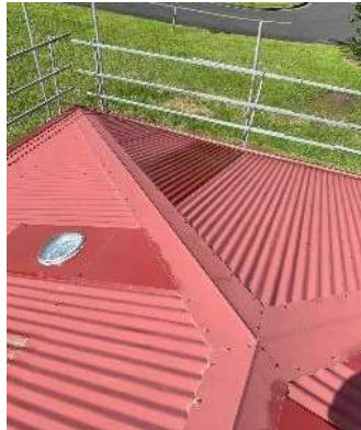
Riverside Park Toilets
