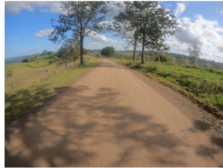
Cross Road – grading works
