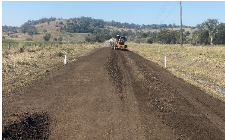
Monaltrie Road – Grading Works
