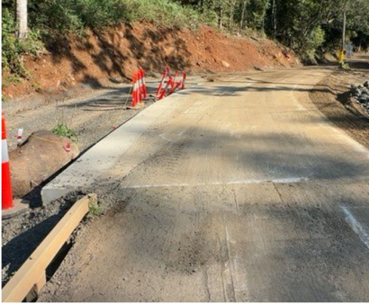
Terania Creek Road – Bridge 2
