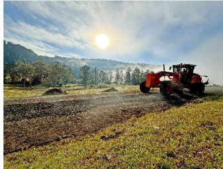
Bice Road – Grading Works
