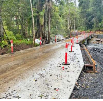
Terania Creek Road – Bridge 2
