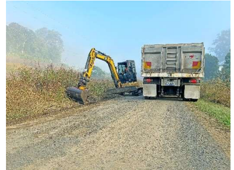
Yeagar Road – Grading Works
