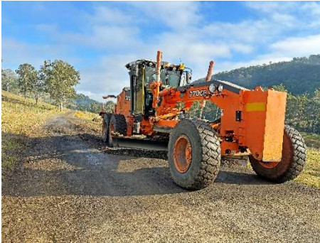
Bice Road – Grading Works
