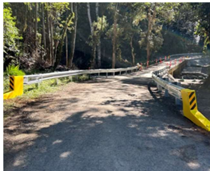
Bridge 3 – Guardrails installed
