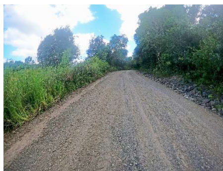
Milgate Road (After)
