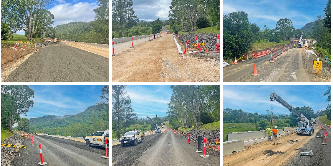
Nimbin Road – Site 4Km (Near Shipway Road) Works
