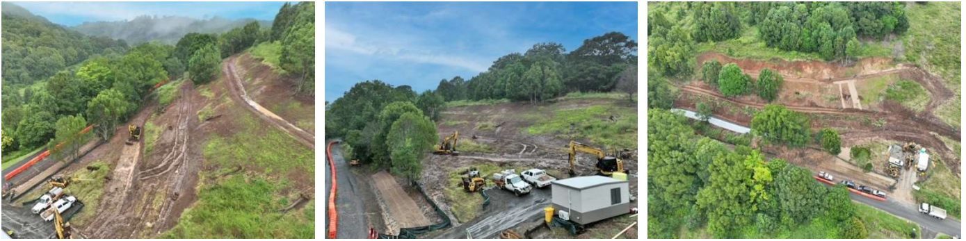
Rosebank Road – Progress Works
