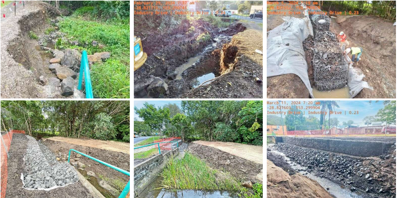
Industry Drive – Before, During and After Works
