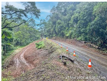
Upper Tuntable Falls Road – Temporary Ramps
