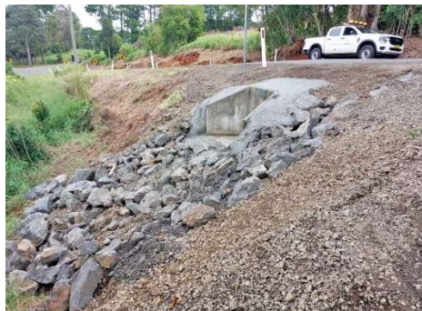
Johnston Road – Culvert Works
