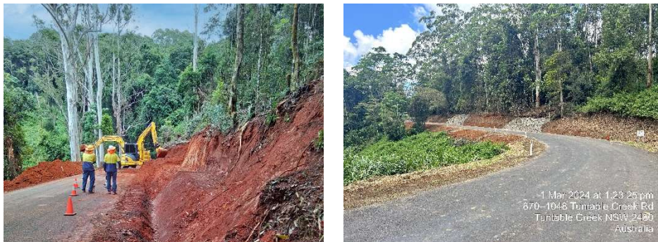
Tunable Creek Road – Progress Photos
