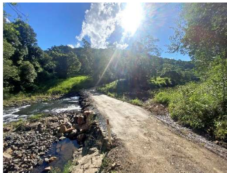
Black Road – Culvert Works
