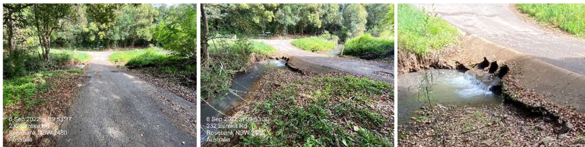
Eureka Road – Culvert
