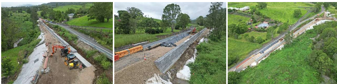
Site 4Km Works
