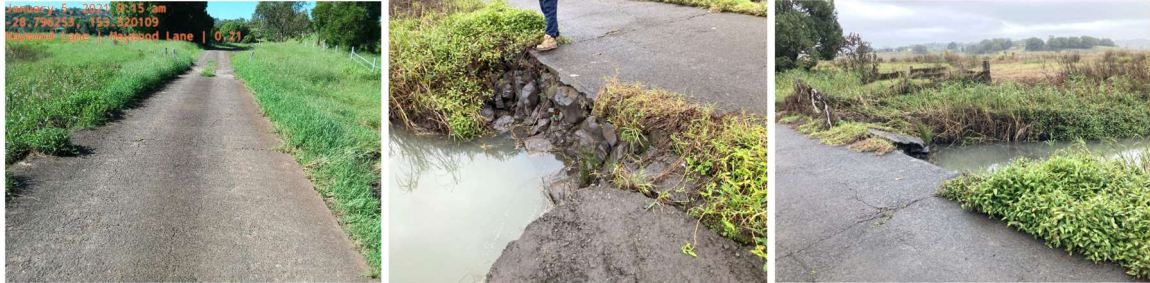
Haywood Lane – Culvert
