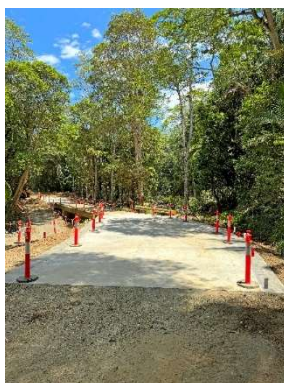
Terania Creek – Bridge 3
