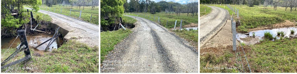
Graham Road – Culvert
