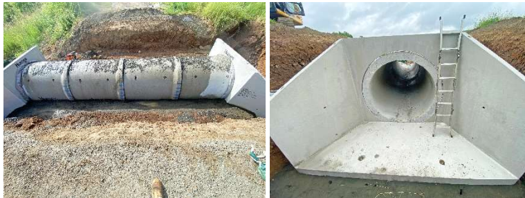
Quilty Road – Completed Works
