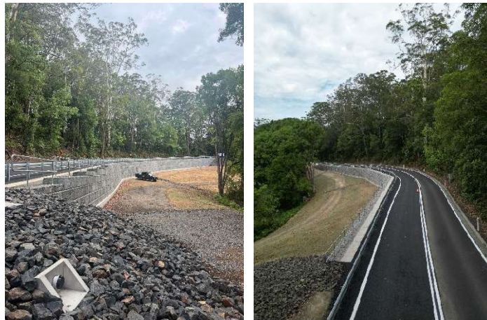
Nimbin Road - Site 1Km Completed Works
