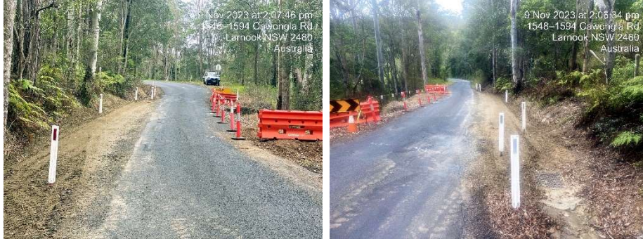
Cawongla Road – Completed Works
