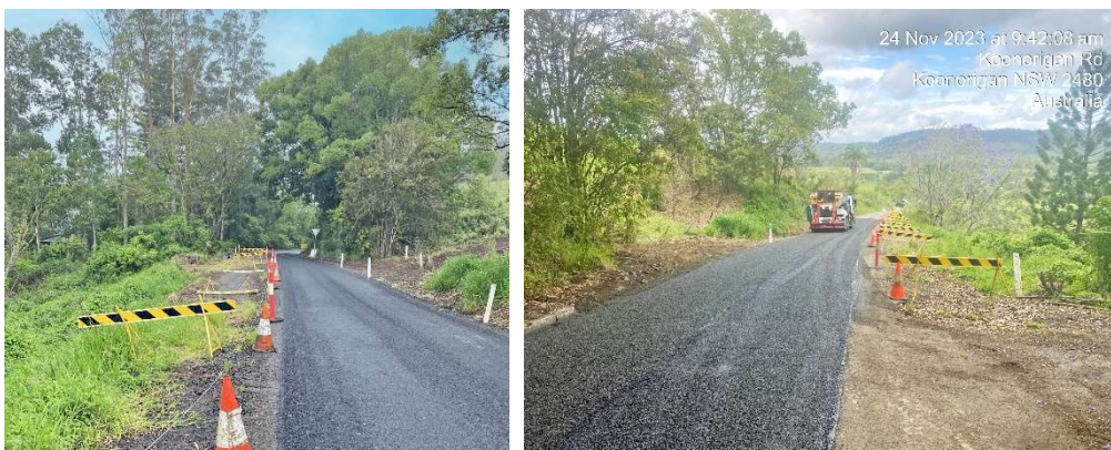
Koonorigan Road – Maintenance Works
