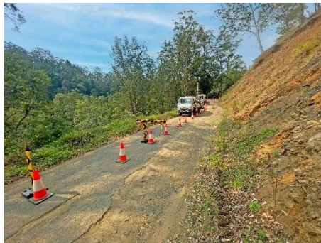
Geotech Drilling on Mountain Top Road
