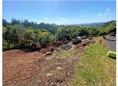
Carabeen Road – During Construction
