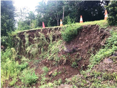
Carabeen Road – Before Works
