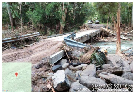
Terania Creek Road (Bridge 3)
