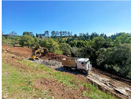
Carabeen Road – During Construction
