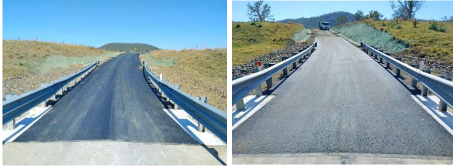
Bungabbee Road Completed Bridge Approaches
