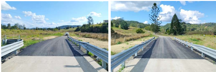
Dudgeon Road Completed Bridge Approaches
