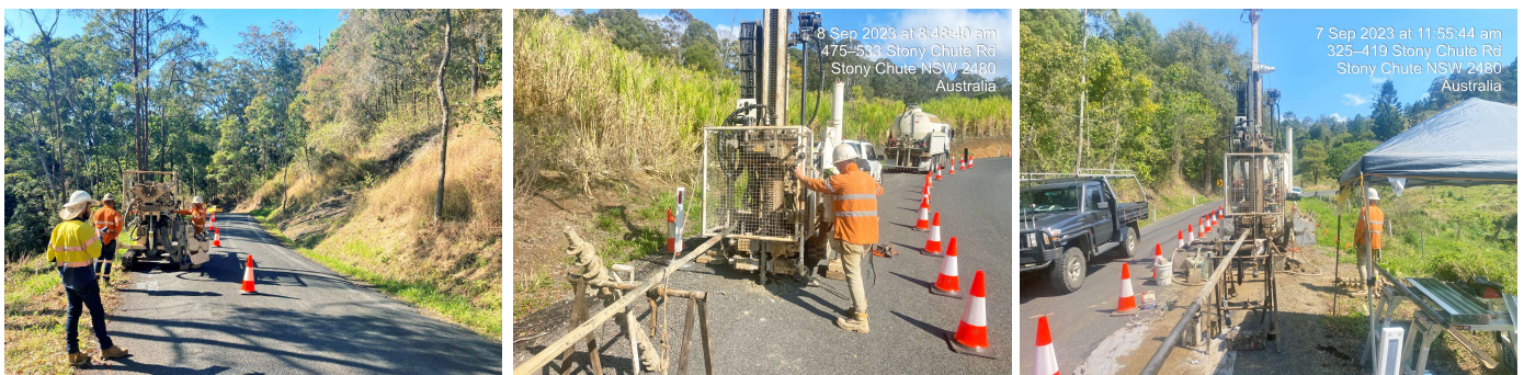
Geotechnical Investigations on Stony Chute Road
