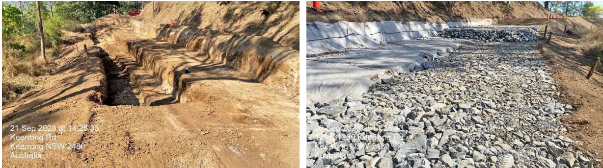
Keerrong Road before and after excavation and drainage rock works
