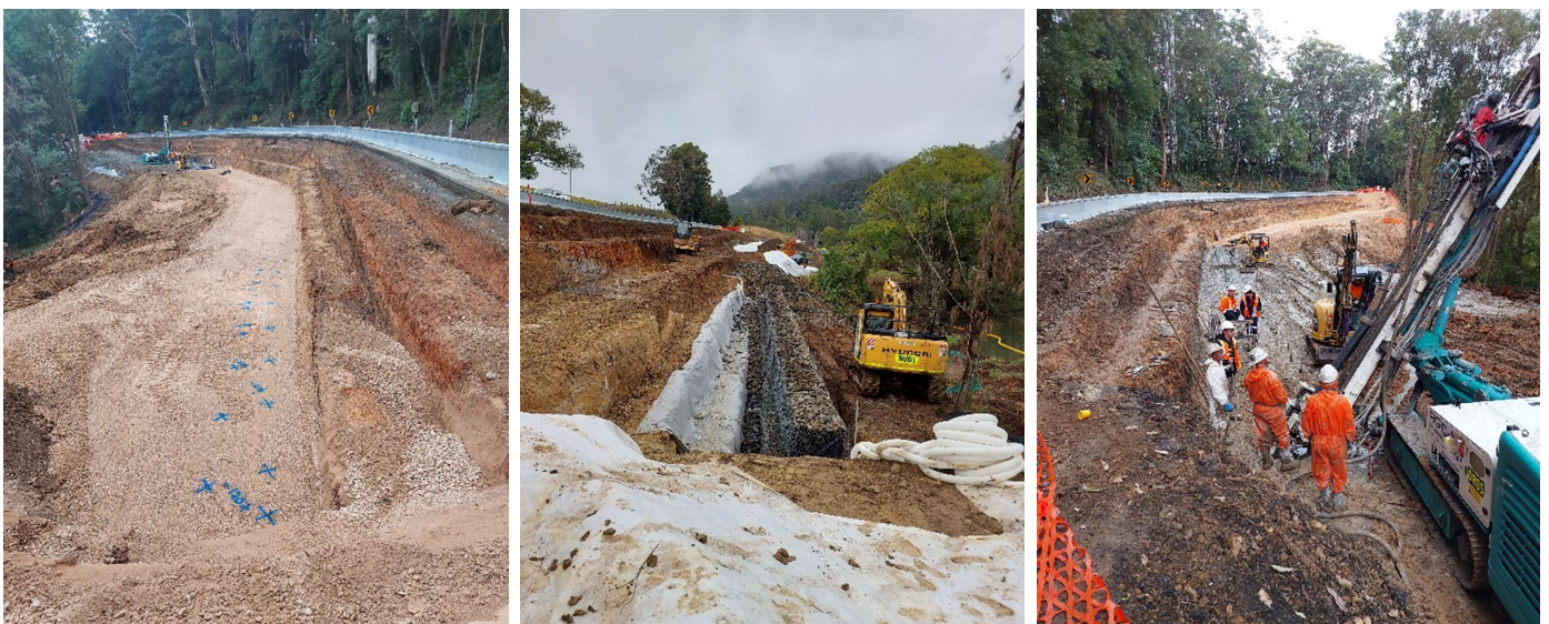
Nimbin Road Works
