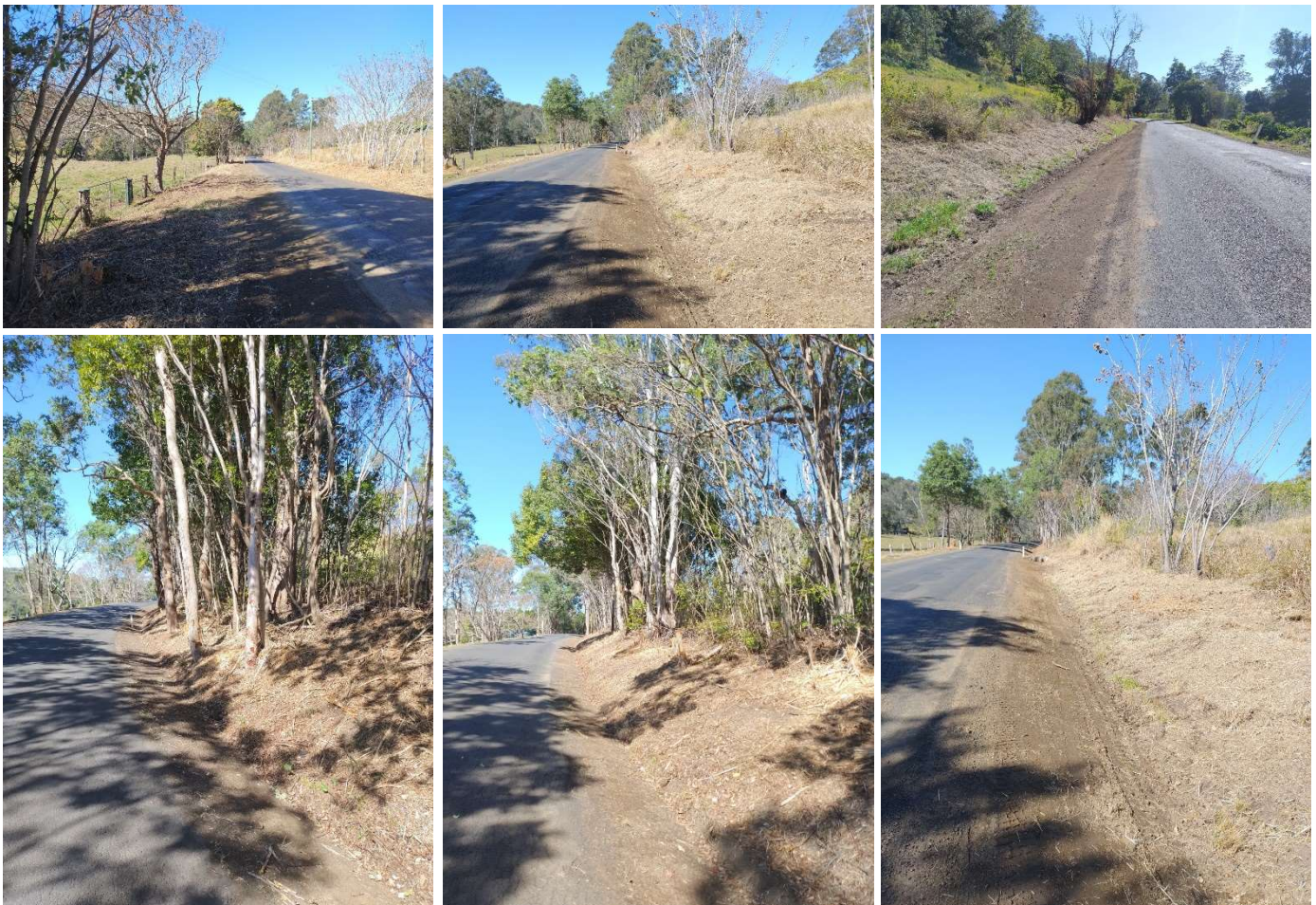
Drainage works on Cawongla Road
