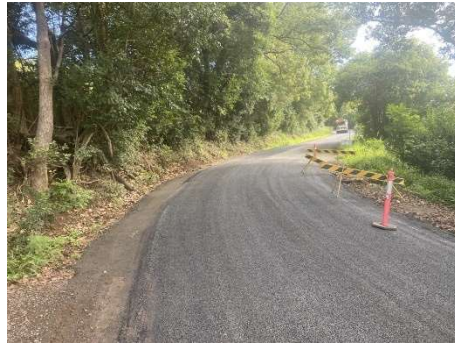
Johnston Road after works
