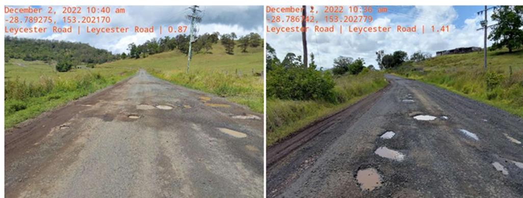
Image: Leycester Road before works
