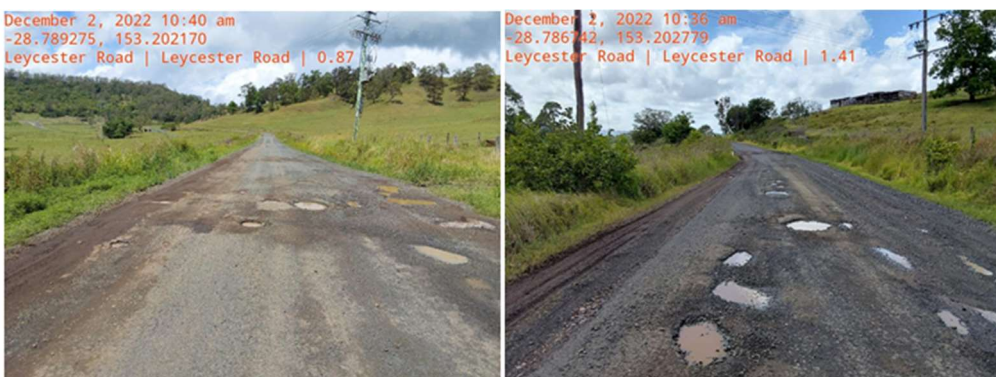
Image: Leycester Road before works
