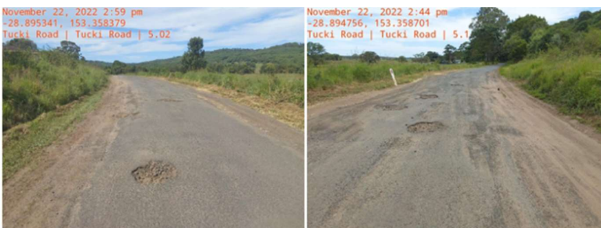
Image: Tucki Road before works
