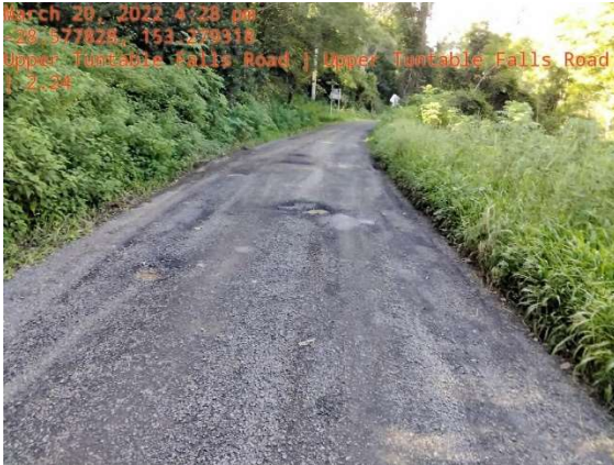
Image: Upper Tuntable Falls Road before works
