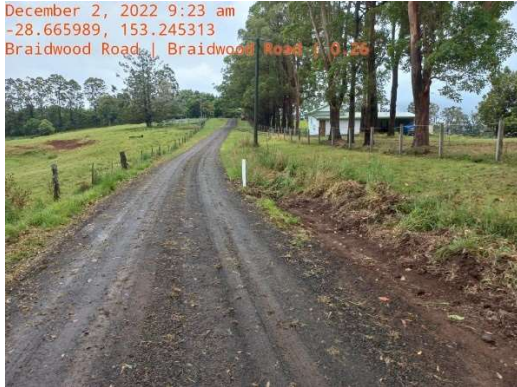
Image: Braidwood Road completed works
