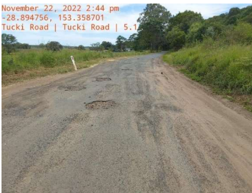
Image: Tucki Road before works image
