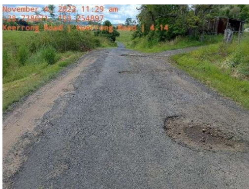
Image: Keerrong Road works
