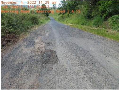
Image: Keerrong Road works
