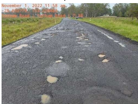
Image 30-32: Tatham Road temporary pavement identified are requiring works
