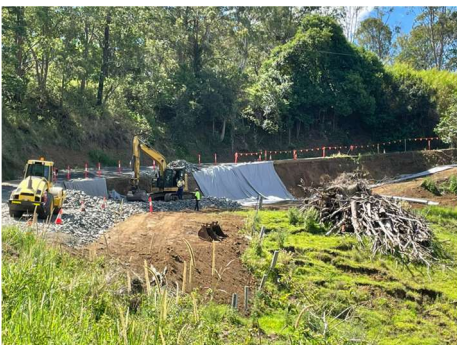
Image 5 & 6: Stoney chute road temporary stabilisation of slip
