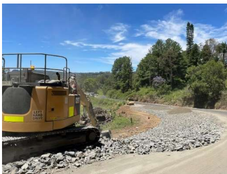
Image 5 & 6: Stoney chute road temporary stabilisation of slip
