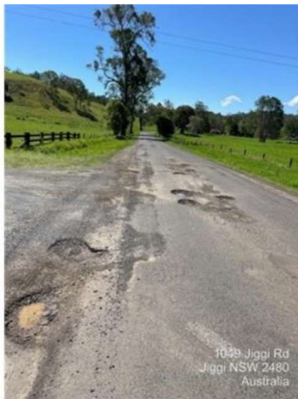
Image 16, 17 & 18: Identified pavement repairs required on Jiggi Road
