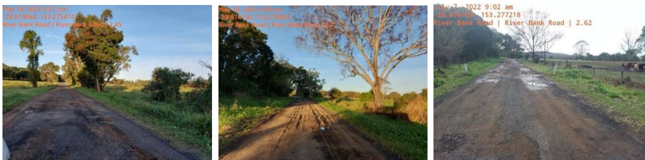
Image 13, 14 & 15: Riverbank Road pavement stabilisation works
