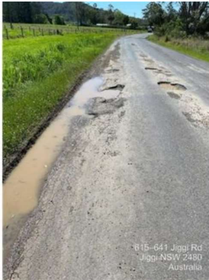
Image 16, 17 & 18: Identified pavement repairs required on Jiggi Road
