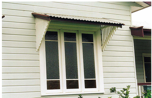
Example of casement windows with long narrow proportions.
