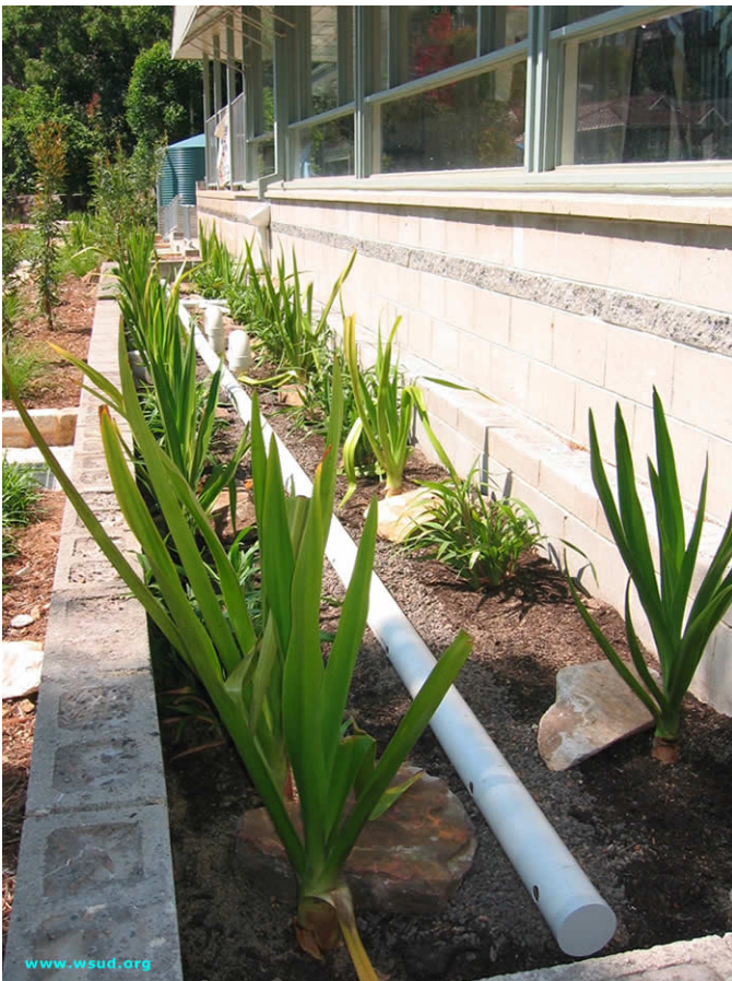
Plate 1.2 Bioretention planter box
