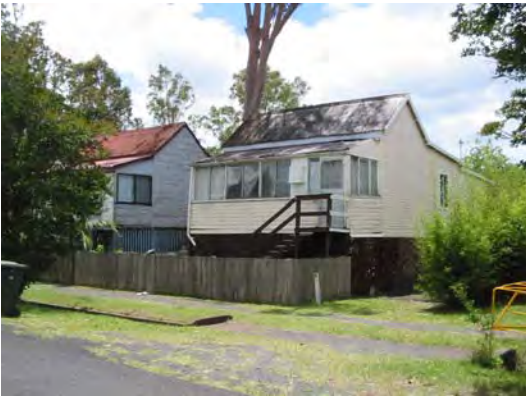
Early cottages in Parkes St
