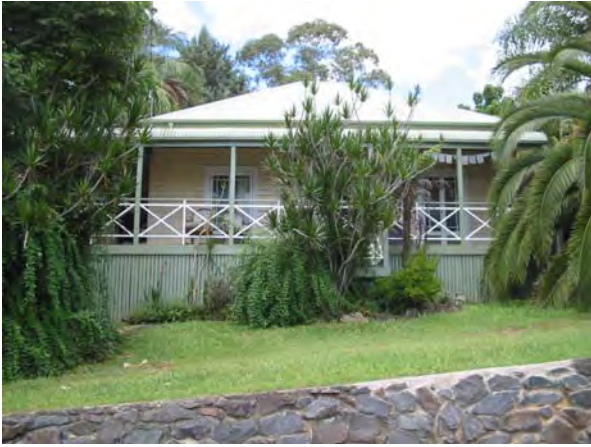
Bullnose verandah with traditional hipped roof to main dwelling. The balustrade may be a later addition.
