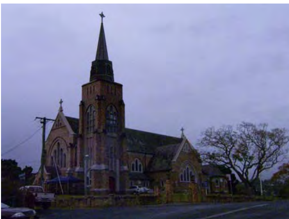
The elevated site gives the magnificent St Andrews Church landmark prominence
