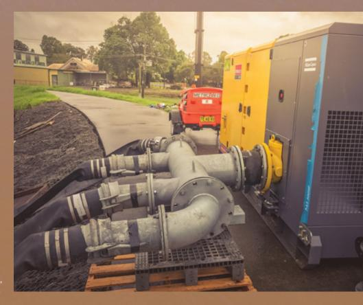
The levels are dictated by the intake levels of the pumps and the depth of water required to operate the pumps without damaging them.
