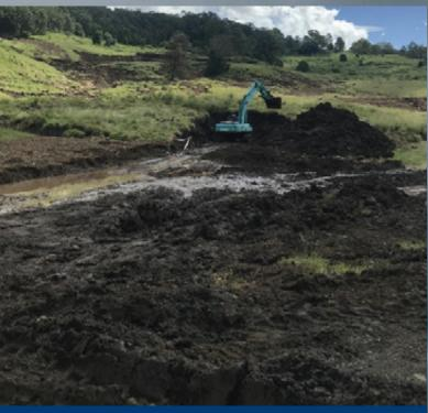
24t excavator clearing landslip over Bice Rd, Leycester
