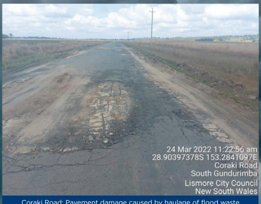
Coraki Road: Pavement damage caused by haulage of flood waste
