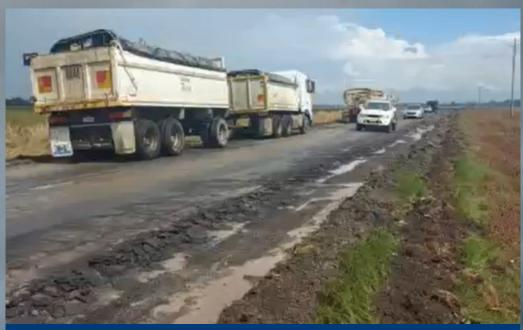
Coraki Road: Pavement damage caused by haulage of flood waste
