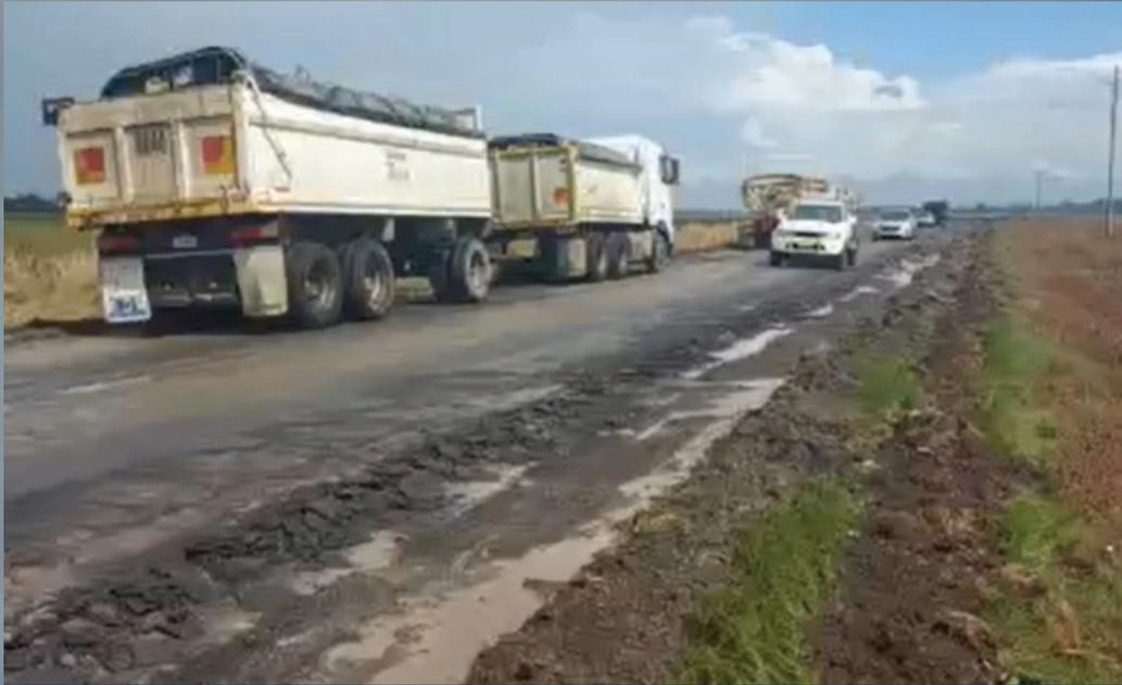
Coraki Road: Pavement damage caused by haulage of flood waste
