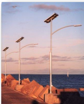
Figure 65: Examples of solar street lighting
