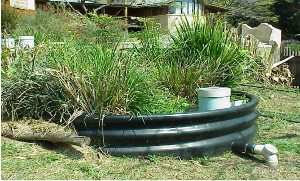
Plate 1. Polyethylene Cattle Trough Reed Bed planted with Lomandra hystrix
