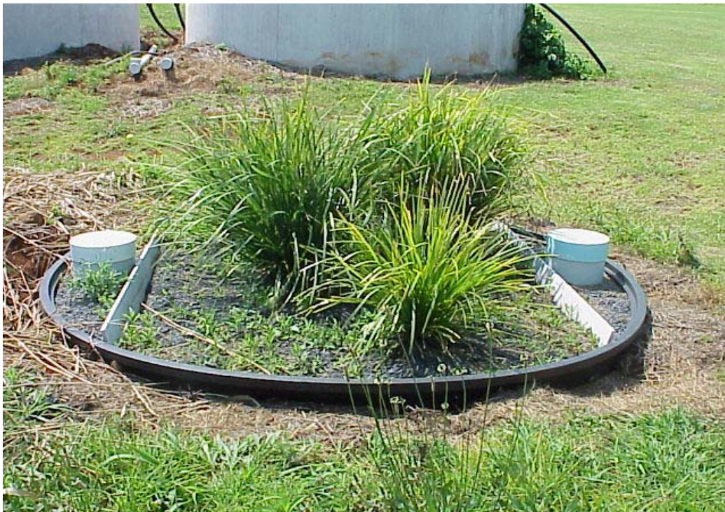
Plate 4. Polyethylene cattle trough planted with Lomandra hystrix . Note the baffle after the inlet structure and before the outlet structure.
