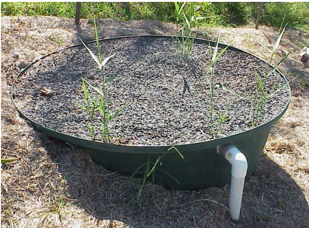
Plate 2. Small Greywater Reed Bed prior to planting with Phragmites australis
