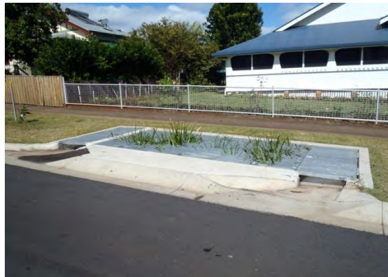
Ecosol raingarden installed on Avondale Avenue, East Lismore - a small vegetated filter designed to provide biological treatment of stormwater run-off at the road kerb side
