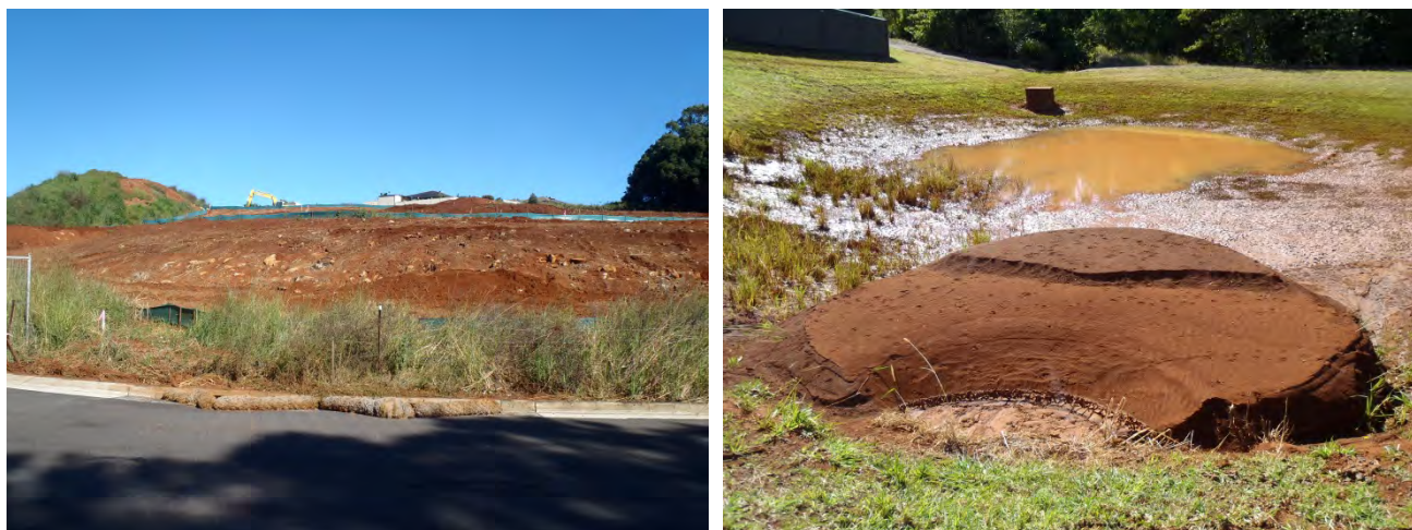
Figure 13: Exposed soil during housing construction and sediment collected in sedimentation basin downstream of the construction site following significant rainfall (May 2015)
