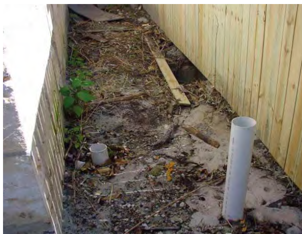
Structures including fences should be clear of field gully inlets. Suitable landscaping along with grid tops to inlets and regular maintenance assists with filtration into council's stormwater system.
