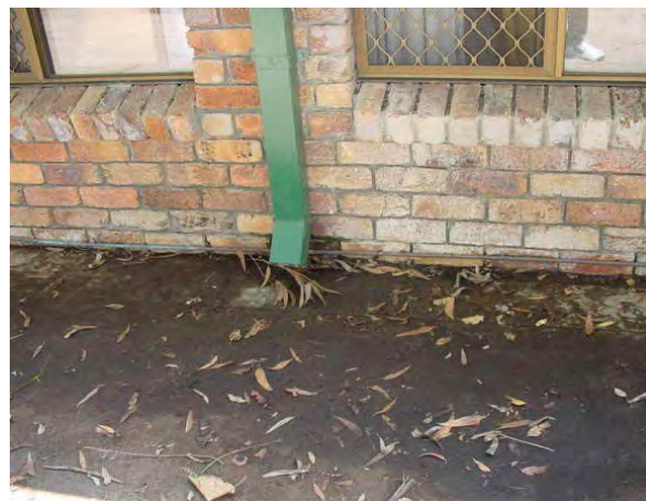
Roof gutters not connected to approved stormwater outlets can cause damage to your property and neighbouring properties
