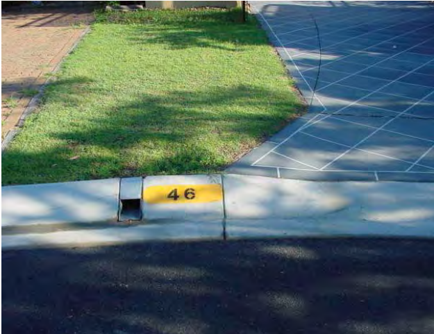
Approved outlet to Council's stormwater drainage system.
