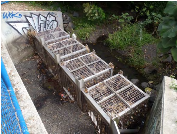
Gas Works Creek – restoration, head wall reconstruction and installation of litter cages
