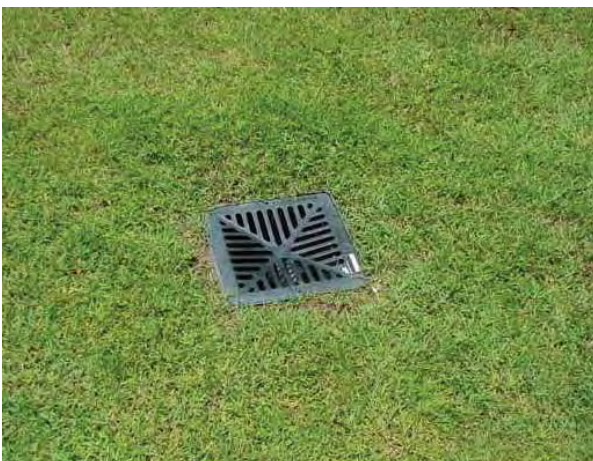
Stormwater gully pit landscaped to collect surface water.
