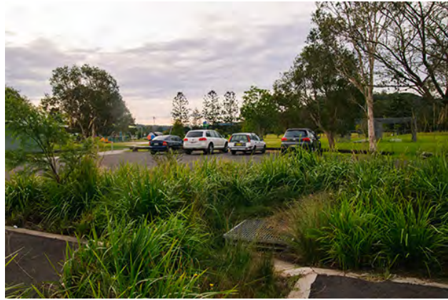
Bio-retention system at Nesbitt Park carpark, South Lismore. Runoff from the new carpark drains into gardens where the soil microbes and plants treat pollutants including hydro-carbons. Source: LCC website
