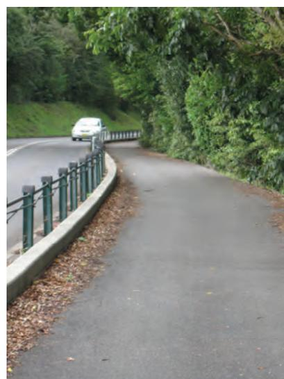
The Rotary Drive route constructed with Brifen safety fencing separating cyclists and pedestrians from the traffic lanes
