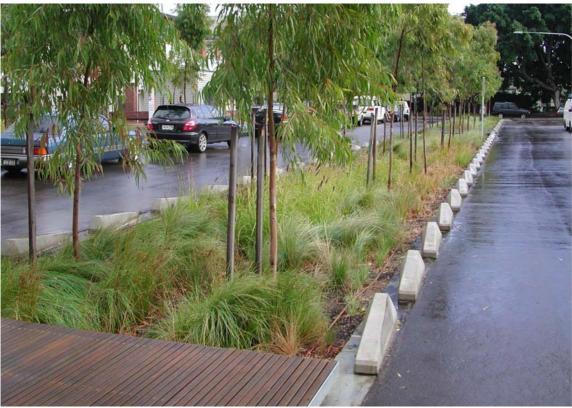
Plate 1.4 Bioretention swale in the centre median of a road
