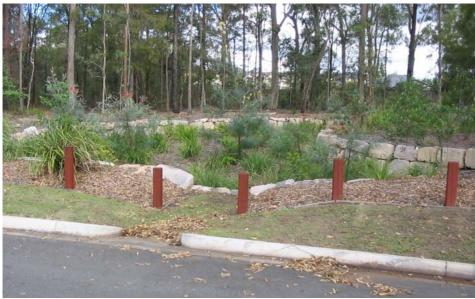
Plate 1.3 Bioretention basin with rock wall perimeter
