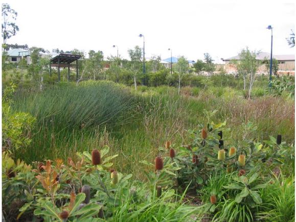
Plate 1.7 Constructed stormwater wetland in a residential setting
