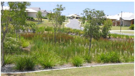
Plate 1.1 Bioretention basin in a streetscape setting
