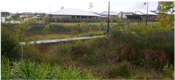
Plate 1.8Constructed stormwater wetland with boardwalkPhoto courtesy of South East Queensland Healthy Waterways Partnership (Water by Design program)
