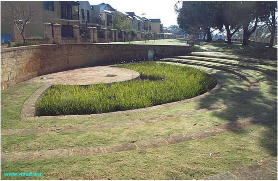
Plate 1.9 Constructed stormwater wetland in urban park setting Photo courtesy of Sydney Metropolitan Catchment Management Authority (Water Sensitive Urban Design in Sydney program)
